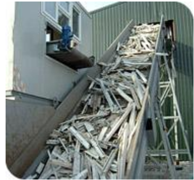
3. Waste entering the processing plant.
